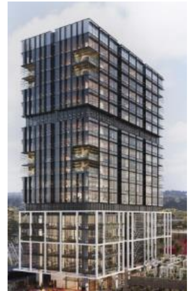
The proposed tower – taller than the towers at the Delhi Rd/Epping Rd junction
